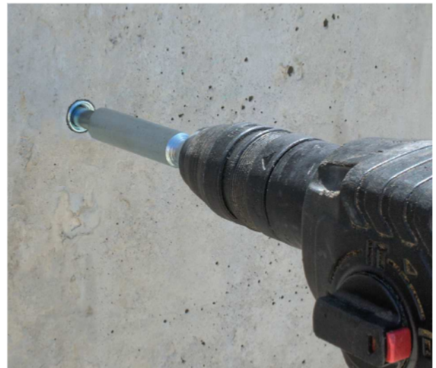
Anchor being set with SDS setting tool.
