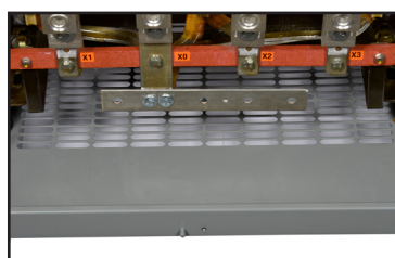
Bottom cable entry area where applicable
