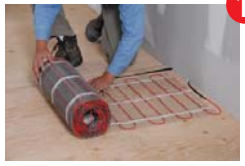
Unroll the self-adhesive mat onto the floor
