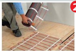
Cut the mesh to turn Never Cut the RED Cable
