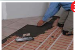
Install tile / floor coverings
