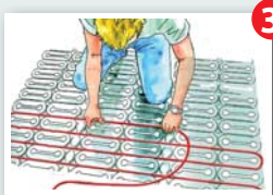
Install heating cable in grooves, pressing gently
