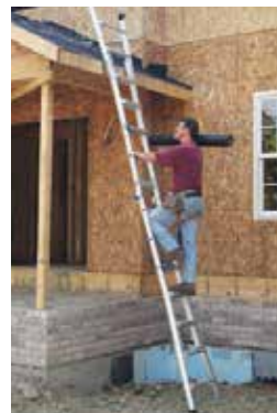
POSITION #3 Extension Ladder
